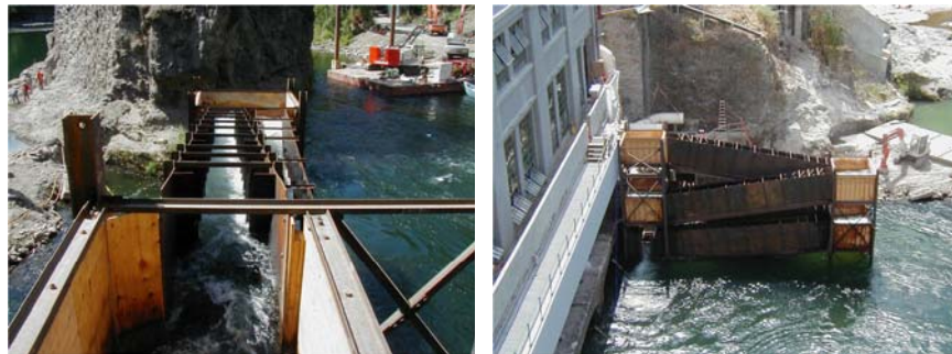
River Mill Temporary Denil Ladder (Photos courtesy of Peter Christenson, R2 Engineering)
