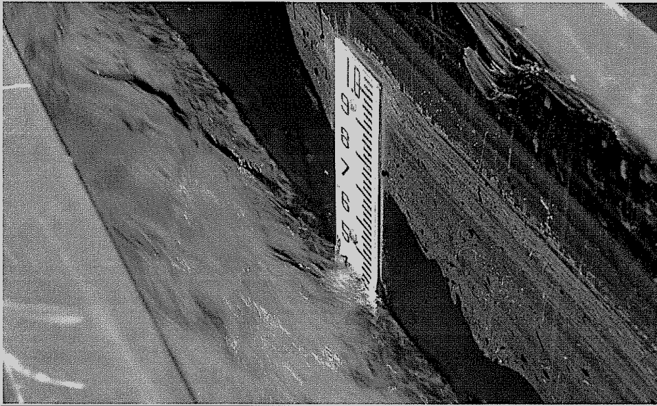
Image 5, middle screen operating water depth
