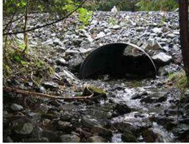
Stream Simulation Culvert
