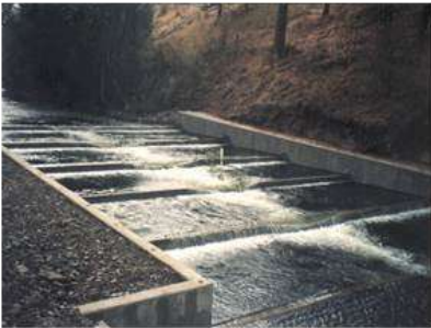
Pool and Weir (full-channel)
